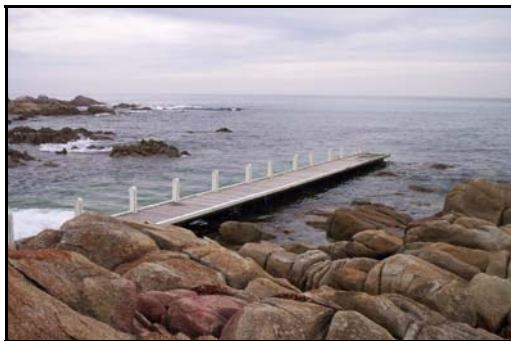
Cape Conran ramp
